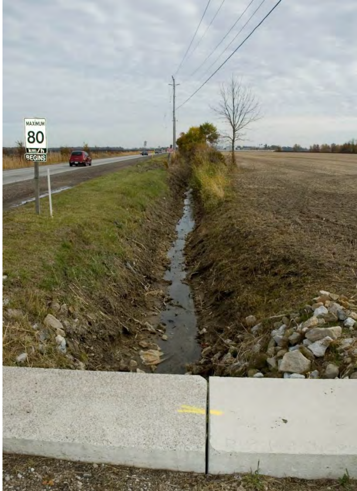
Plate 6: North Townline Drain south of adjacent County Road 42 (October 18 2009).
