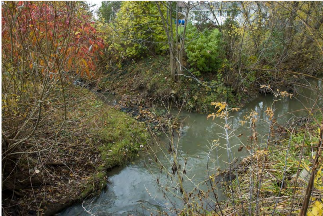
Plate 9. The 8 th Concession Drain (upper left drain) at the confluence with 6 th Concession Drain (Location N42°14.779 W082°56.736).
