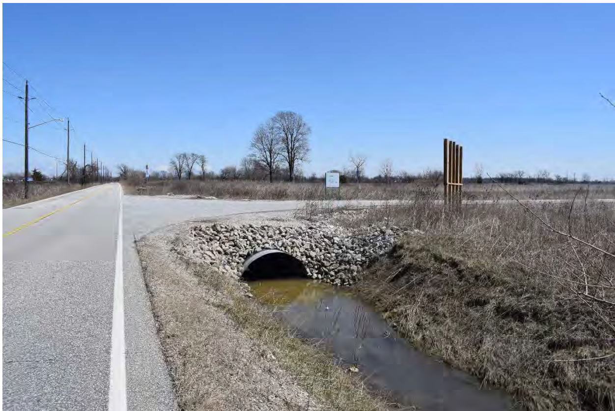
Plate 1: Deep ditch and culvert driveway example on EC Row Avenue East
