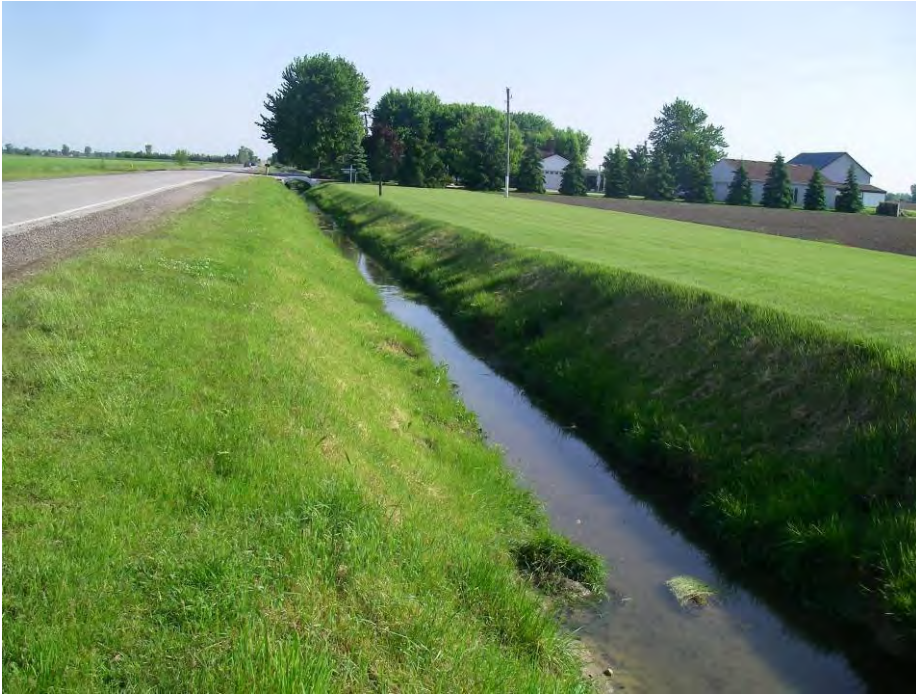
Ninth Concession Drain (NCD-1) Looking upstream from near middle of reach
