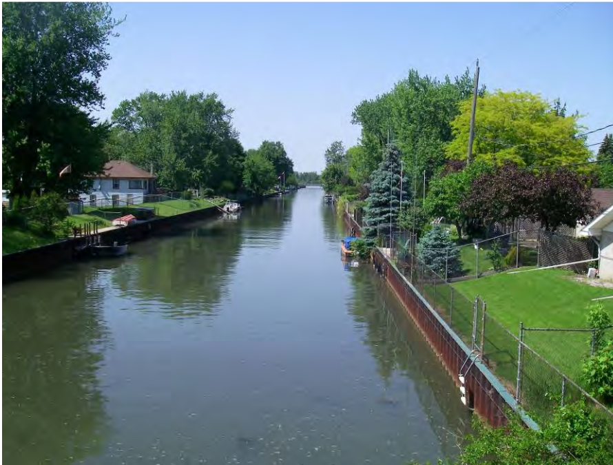
Little River Reach (LR-1) Looking downstream at retaining walls
