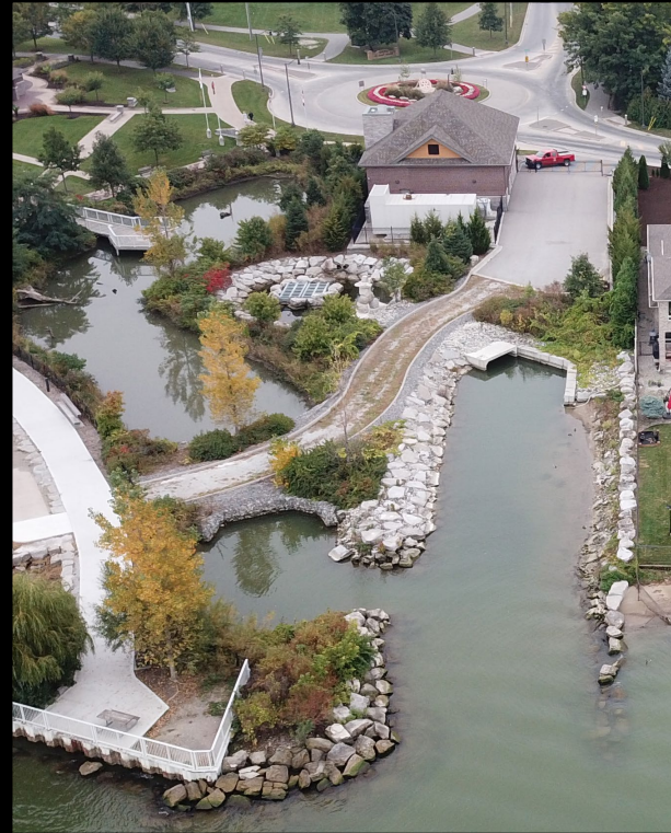
East Townline Drain Pump Station - AFTER
