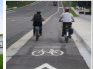
Cycle Track Separated by Mountable Curb, East Gwillimbury
