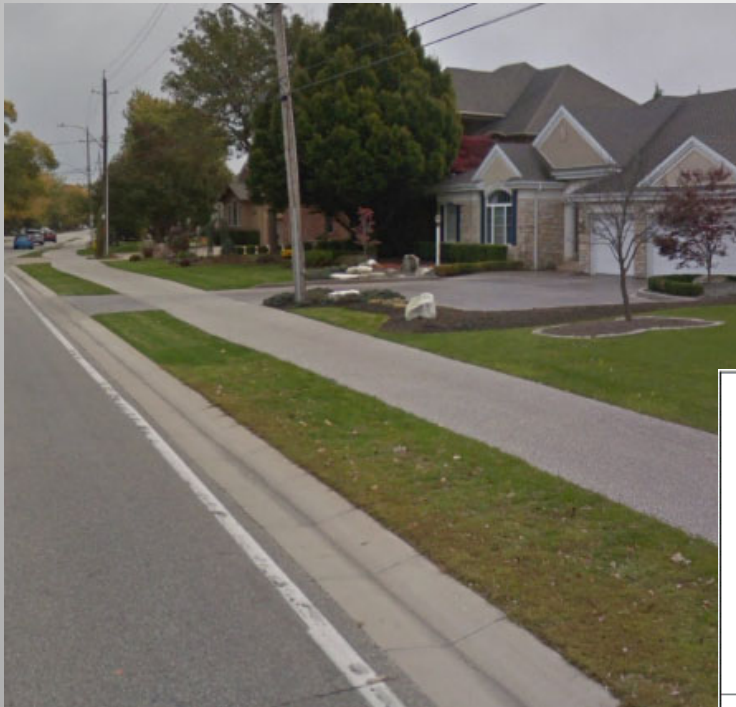
East of Manning Road Multi-Use Trail
