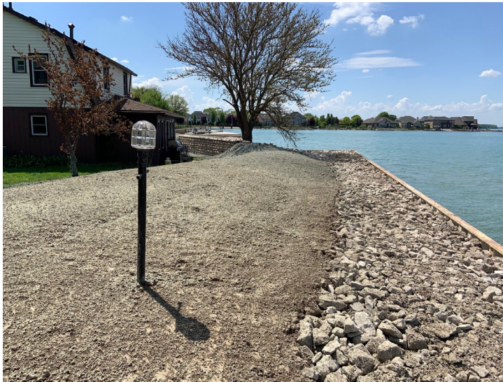
(Figure 2: Image of Clay Berm along Lake St. Clair)
