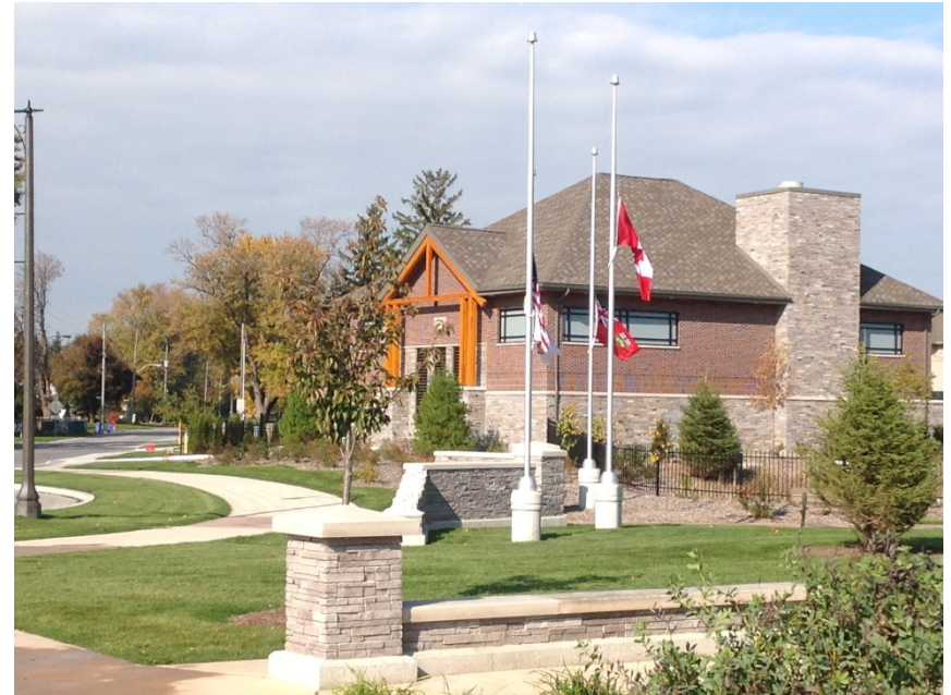
East Townline Drain Pump Station
